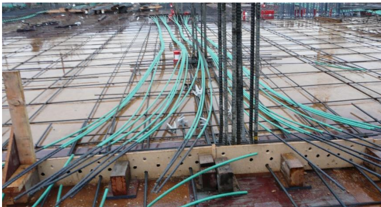
Post-tension cables
