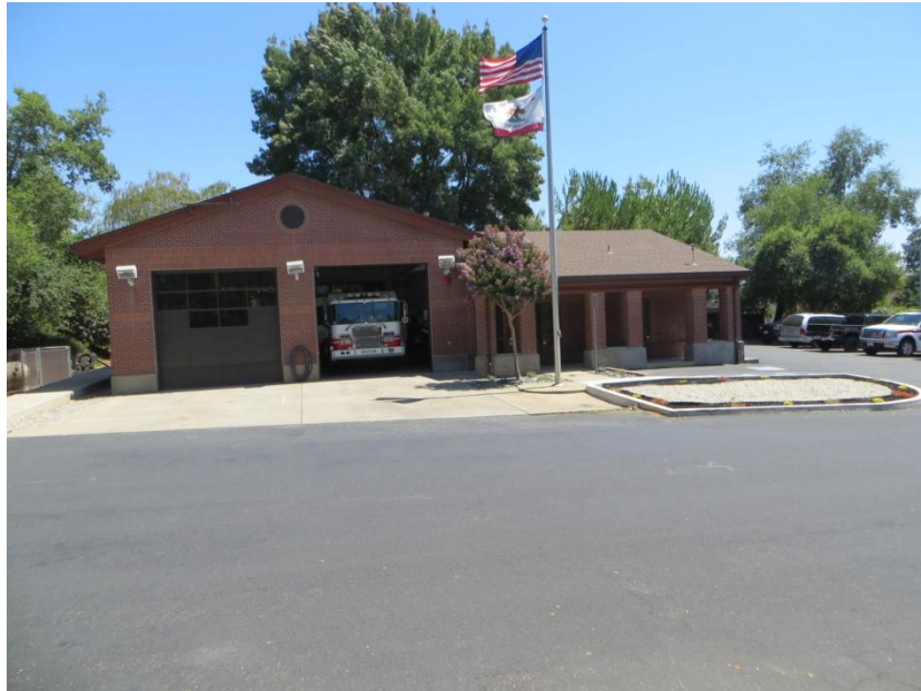
Station 88 (Alhambra Drive; expansion would be on the left side)
