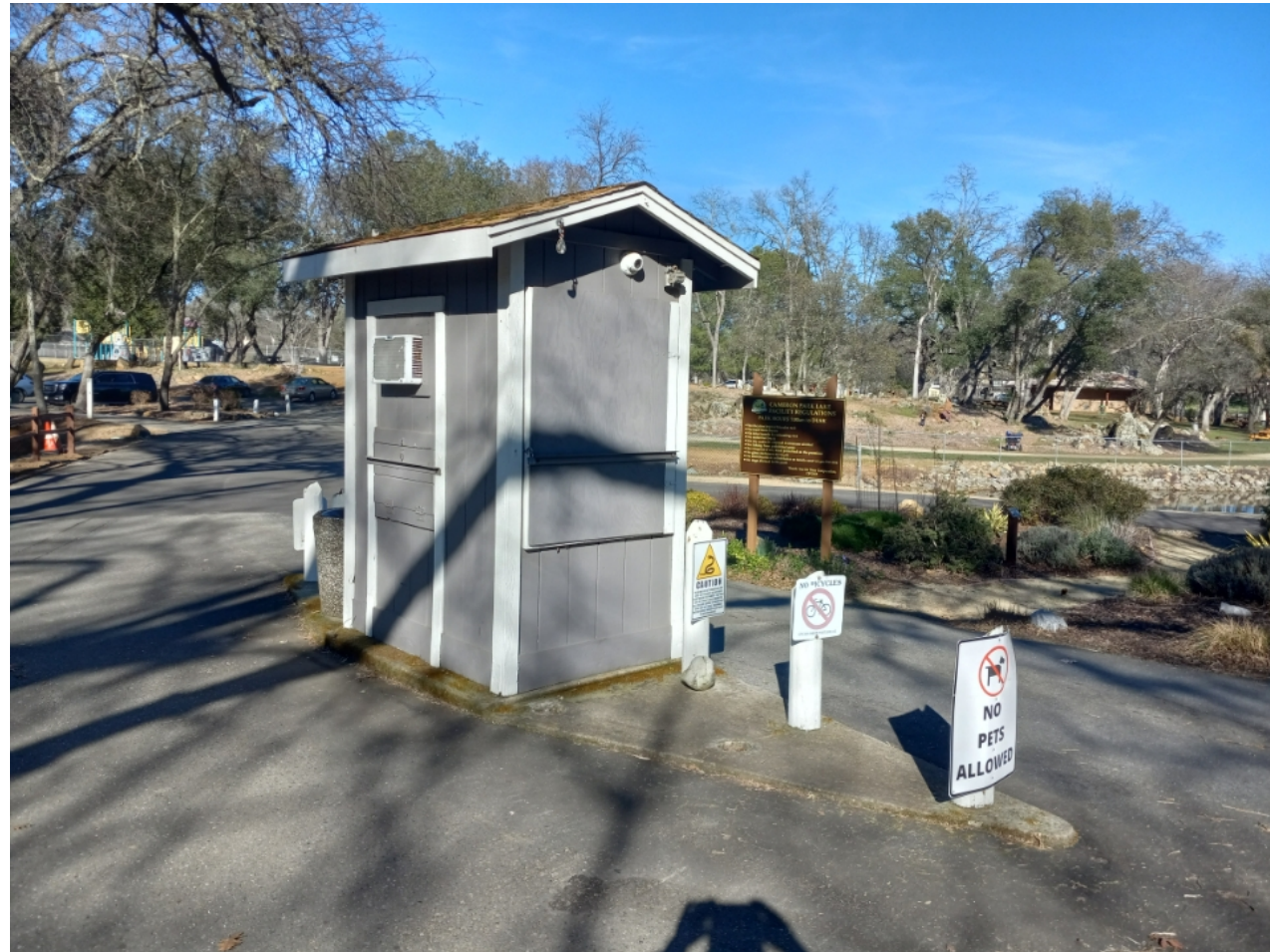
1 GATEHOUSE ENTRANCE - EXISTING CONDITIONS
