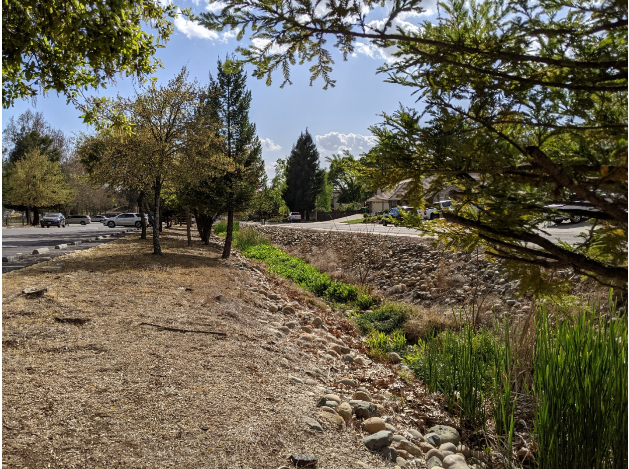
Photograph 4. Drainage on the northwestern side of the park between the parking area and Mira Loma Drive
